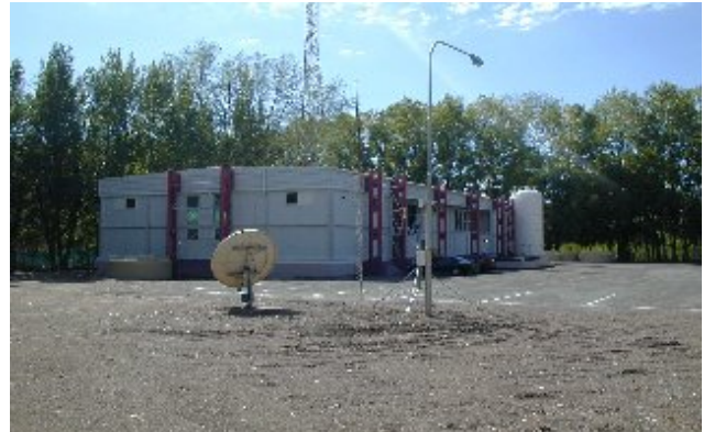
Fig. 7. The assembly building, the internet dish, the 51 m telecommunication tower, and the pure water storage tank.
